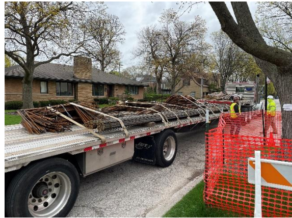
Rebar deliveries for caisson caps and grade beams
