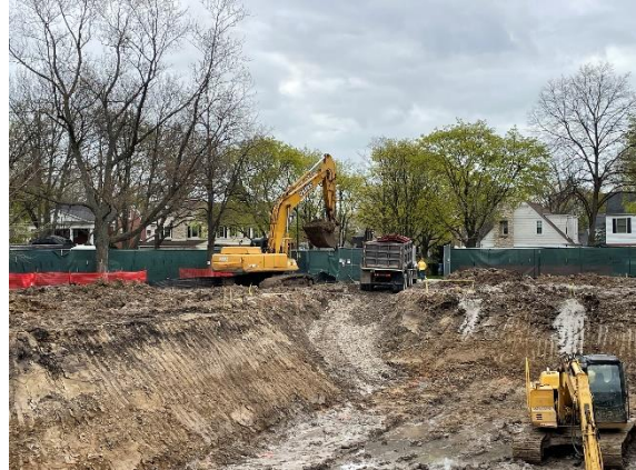
Excavation material haul-off
