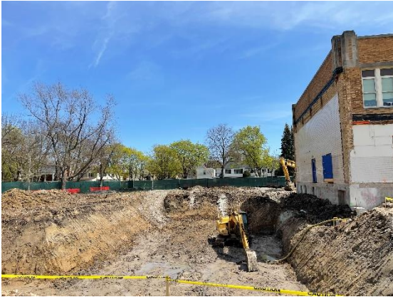
New basement excavation
