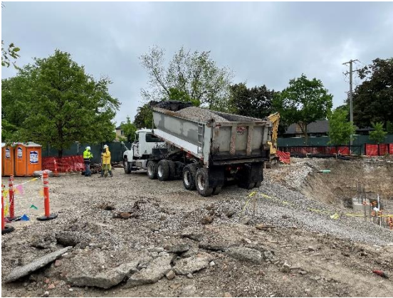
Engineered fill delivery
