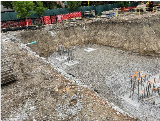
Engineered fill installation at caisson caps
