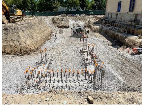
Engineered fill installation at grade beams
