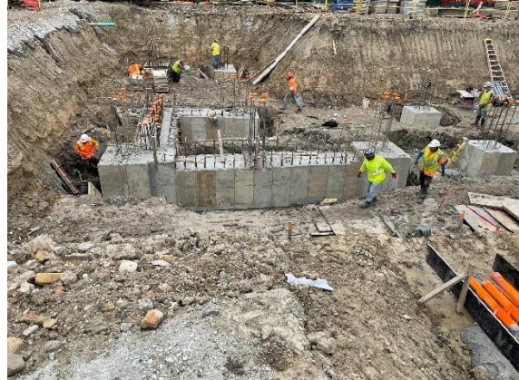
Formwork removal
