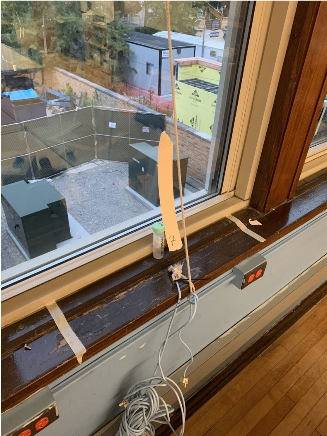
Photo 7: Location 7 – Room 207 – Windowsill (sample GP090622-07A)
