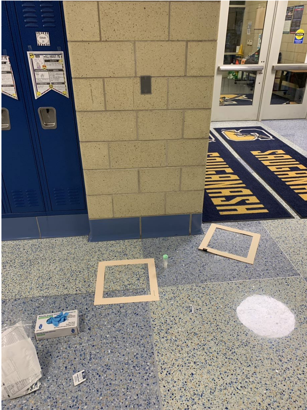
Photo 1: Location 1 – Main Entrance Lobby – Floor (sample GP090622-01A)
