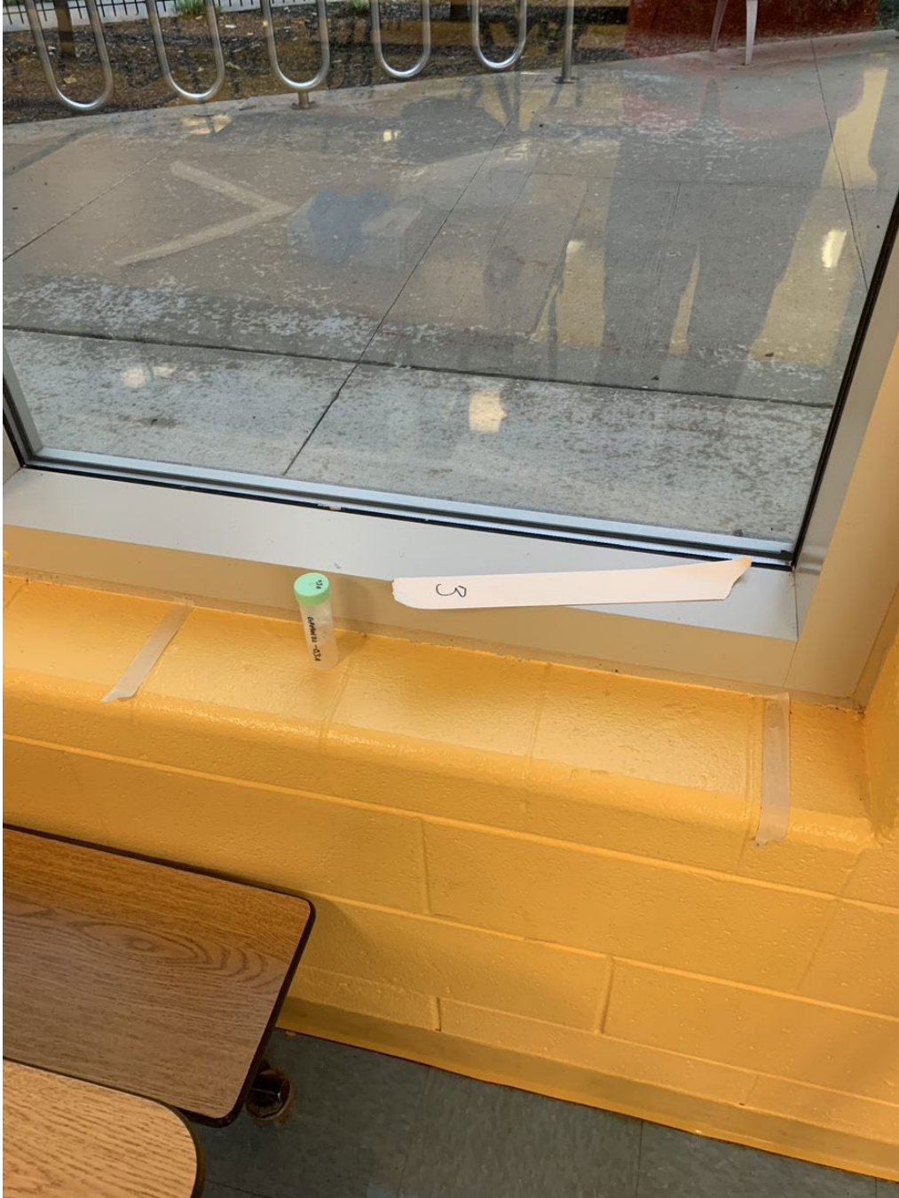
Photo 3: Location 3 – Lunchroom – Window Sill (sample GP090622-03A)
