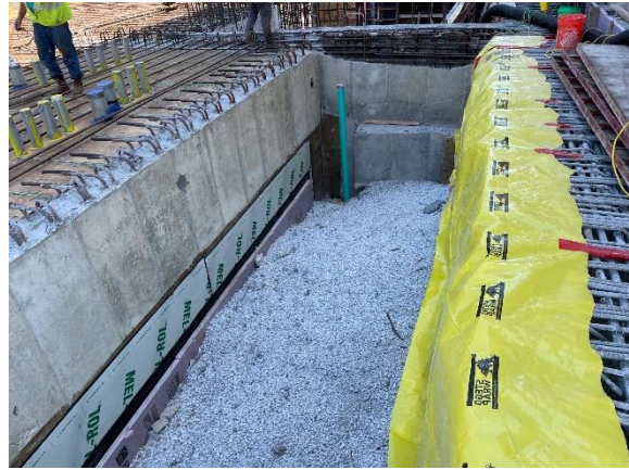
Engineered fill at grade beam # 6
