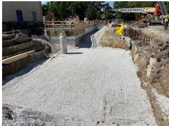
Engineered fill at storm trap
