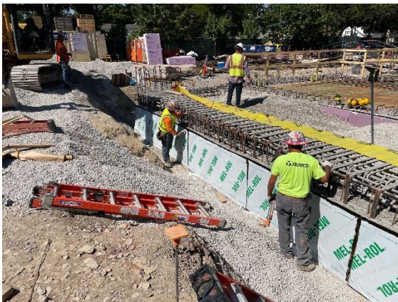
Waterproofing at upper wall of grade beam #6
